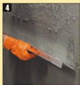
4 Now apply 10-15 mm thk Perlcon OSMOPLAST readymix mortar and match the adjacent plaster surfaces
