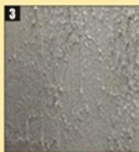
3 First apply an plaster under coat of 6-8 mm using perlcon " SANDFREE " ready mix plaster mortar and allow it dry for 2-3 days
